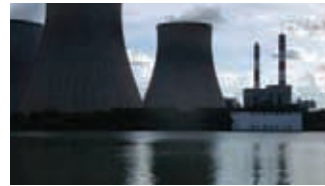
Rayalaseema Thermal Power Project comprises of Stage-I ( 2X210MW ) Stage-II ( 2X210MW ) Stage-III ( 1X210MW ) Stage-IV ( 1X600MW )
